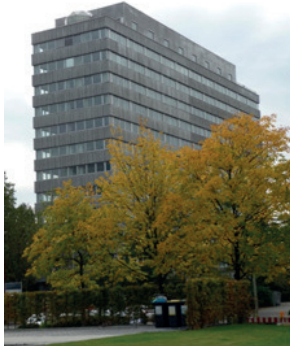
Existing building in present condition
